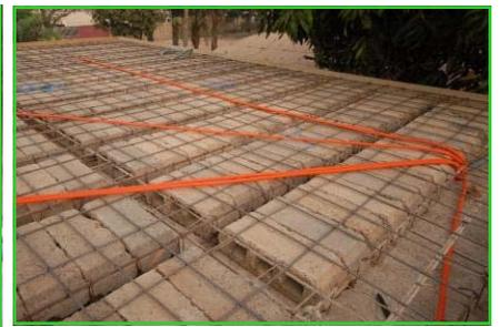
*First the braces go in, then rebar and blocks. After this they poured the concrete and the floor was complete!*
