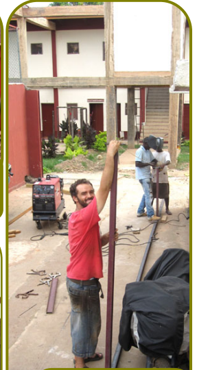
Measuring and welding one of the five solar panel supports
