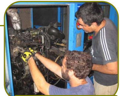
Repairing our diesel generator
