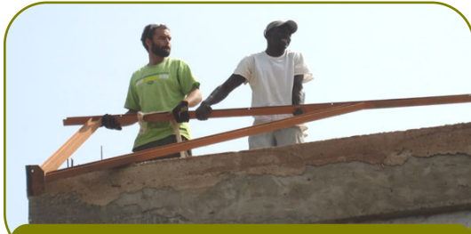
Jason and Nilton pulling the giant steel solar panel support over the top of the controller room
