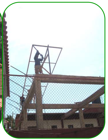
Nothing like welding in the hot African sun ☺
