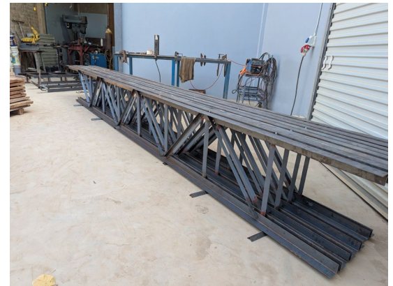
Trusses are starting to stack up, waiting for paint!
